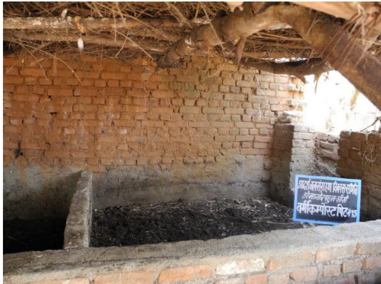
Vermi-compost facility at Gaushala
