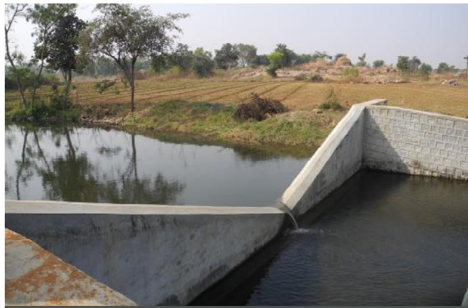
Check dam at Dhikoli
